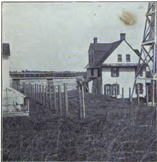
22.—House twenty-four feet wide; posts set and shed at north end built first.
